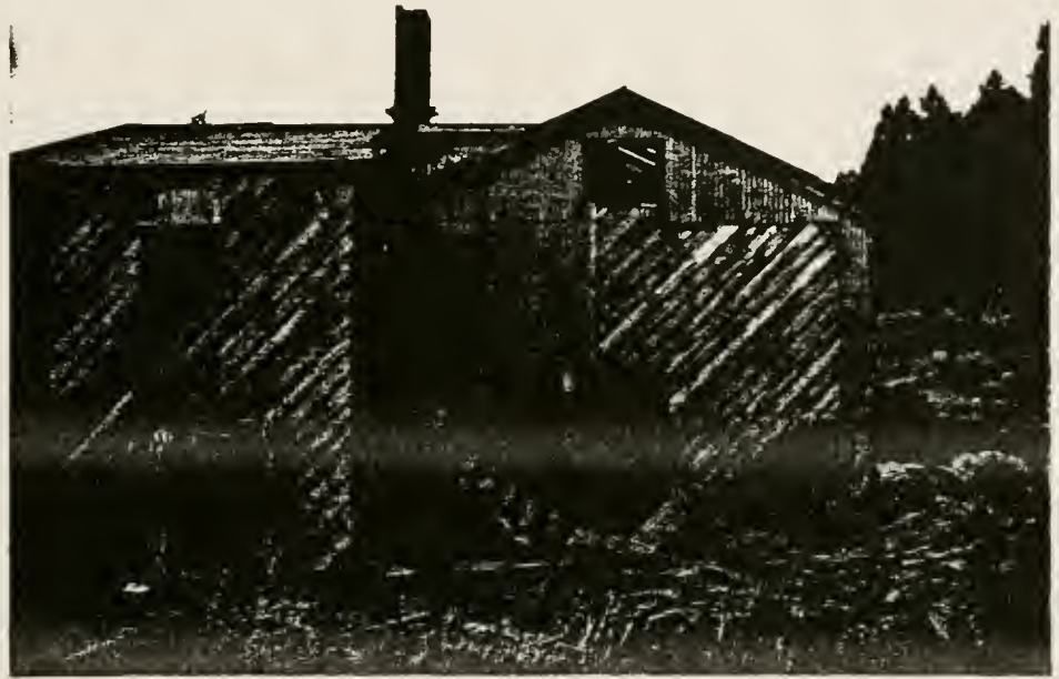
Figure 138. Dry house (structure #50), north view.
